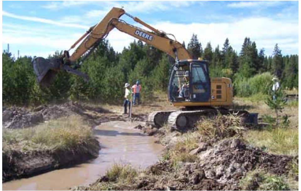
Rebuilding a stream channel to restore connectivity for bull trout, made possible by CFLR. © Craig Bienz
